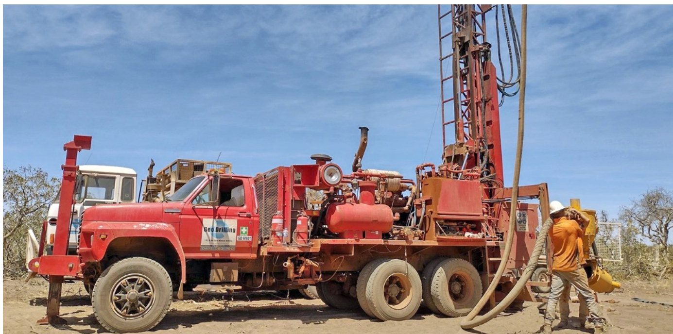
Figure 1 Drilling rig setting up on the first drill collar of the Benmara Project September 2021
